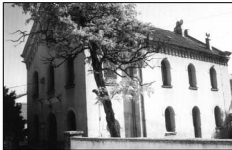
The exterior of the Ashkenazi temple today.
