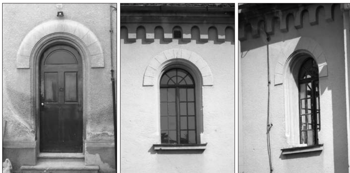
64. Door leading to the gallery, 65, 66. Windows on the first floor
