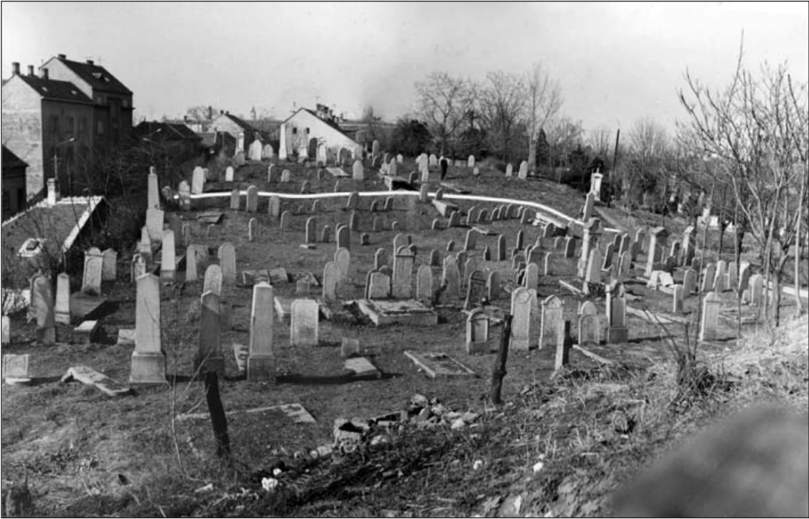
76a. Destroyed part of the cemetery, 1974
